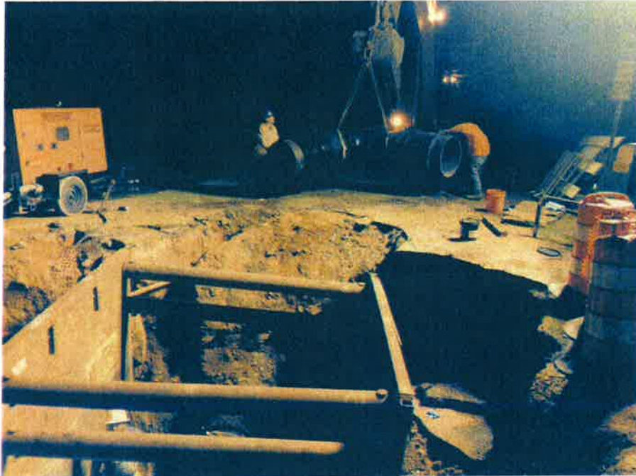
NEW 30" 90 DEGREE BEND AND PIPE READY FOR INSTALLATIO
