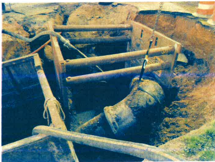
30" FORCE MAIN REMOVAL
