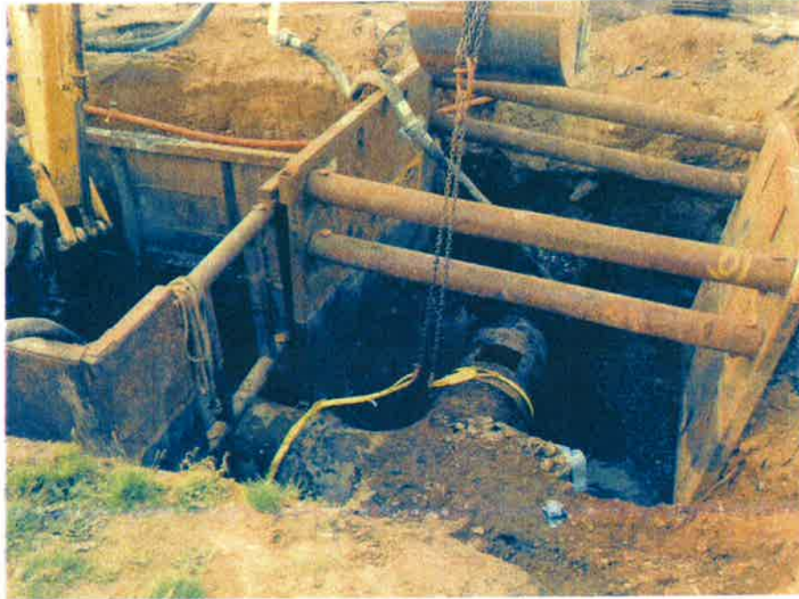
EXISTING 30" FORCE MAIN READY TO BE REMOVED
