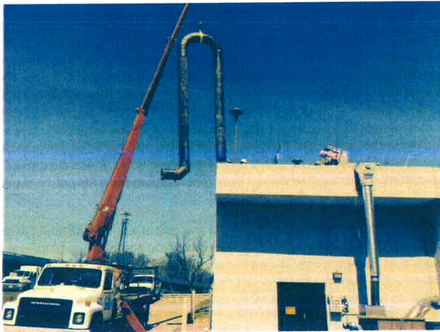
TEMPORAY FORCE MAIN DISCHARGE INSTALLATION AT SCWWTP HEADWORKS
